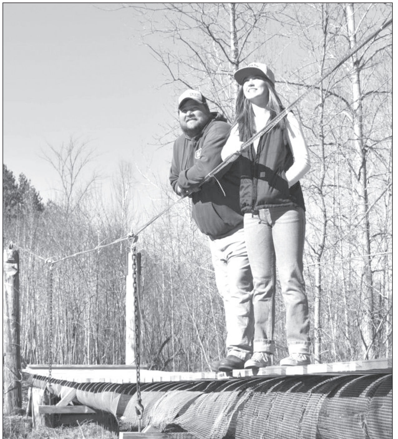
Justin “Buzz” Massie and his 15-year-old daughter, Dakota, look off the 75-foot suspension bridge they constructed last year over the Sturgeon River on their property in Foster City. They built the structure, which Buzz Massie designed, as an easier connection to a nearby ATV trail. (Iron Mountain Daily News photo)
