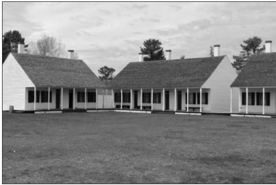
Among major projects scheduled for Fort Wilkins State Historical Park this summer is replacing the roofs of the three officers' barracks. (Daily Mining Gazette photo)
